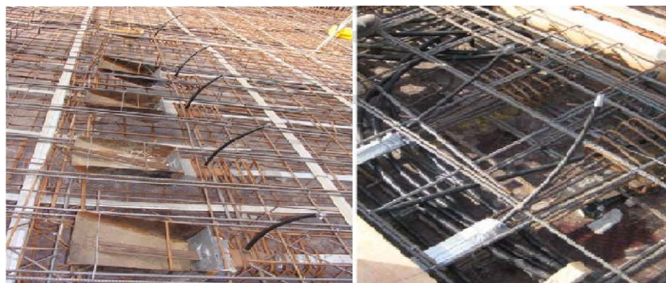
Above—Pan End Grout Tube Above—Dead End Tube (Fig-16)
