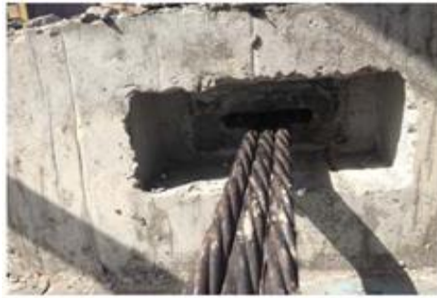
Above-Anchor recess removal (Fig-20)
