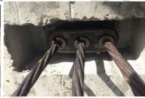
Above-Stressing block installation (Fig-21)
