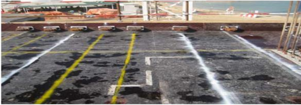
Marking of Tendon Locations (Fig 04)
