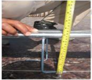
Right-Checking of Tendon Profile (Fig-8)
