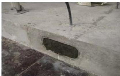
Completed End Stressing Infill (Fig-27)
